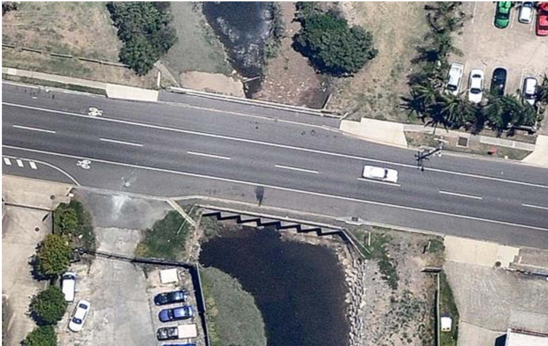
Zillmere Road aerial view
