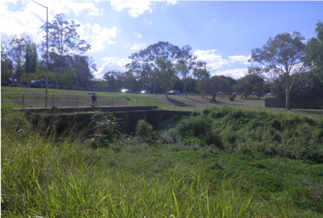
Culverts looking upstream
