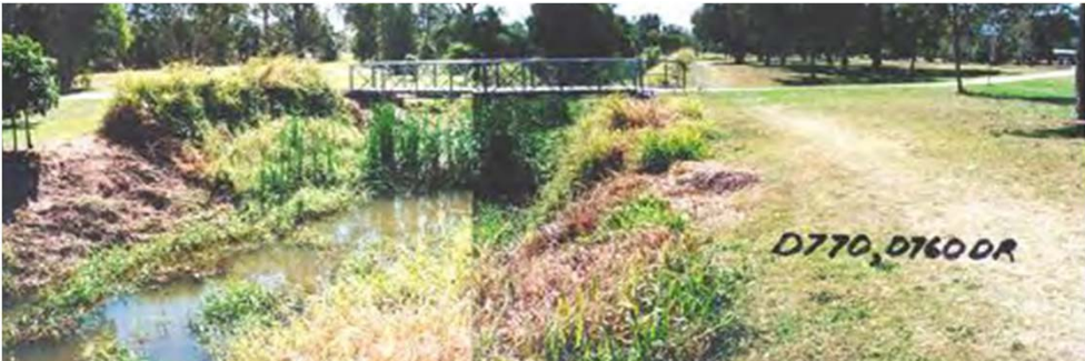
Huxtable Park footbridge
