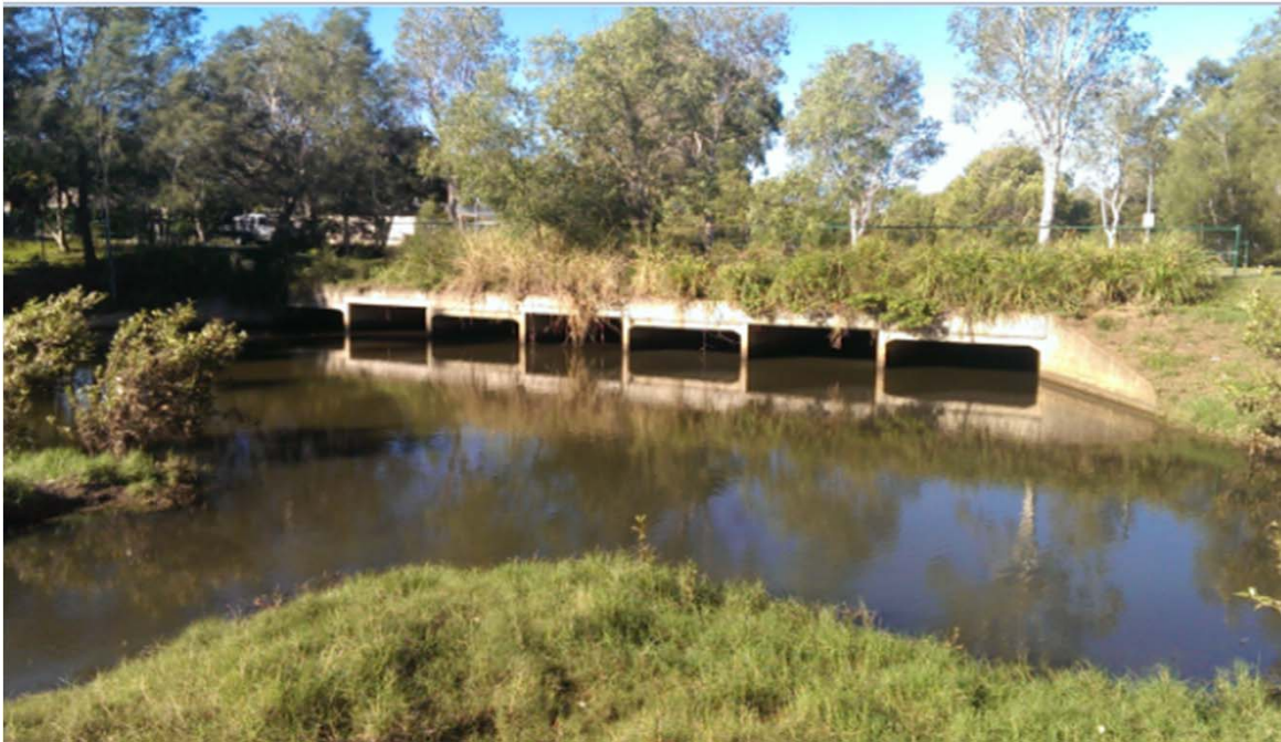
College Way looking downstream
