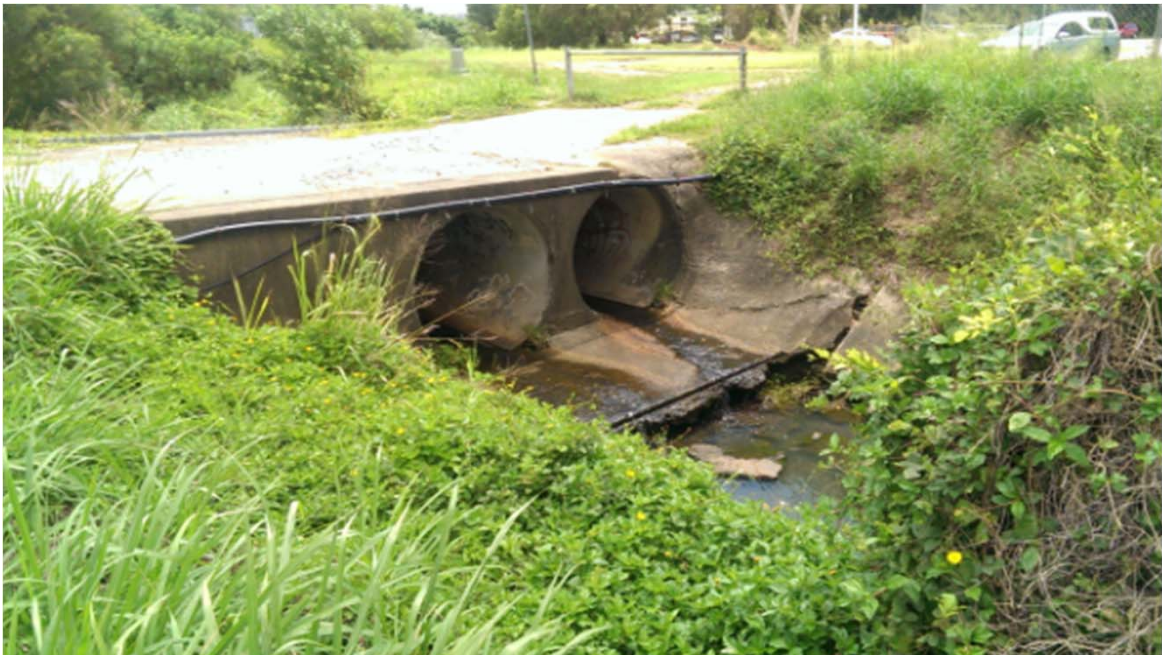
Culvert looking downstream
