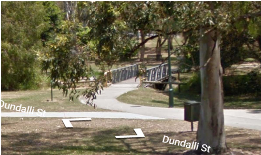
Huxtable Park footbridge looking upstream
