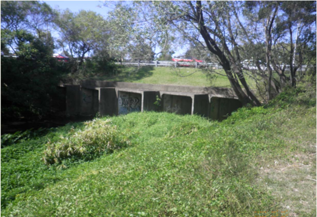
Culverts looking downstream
