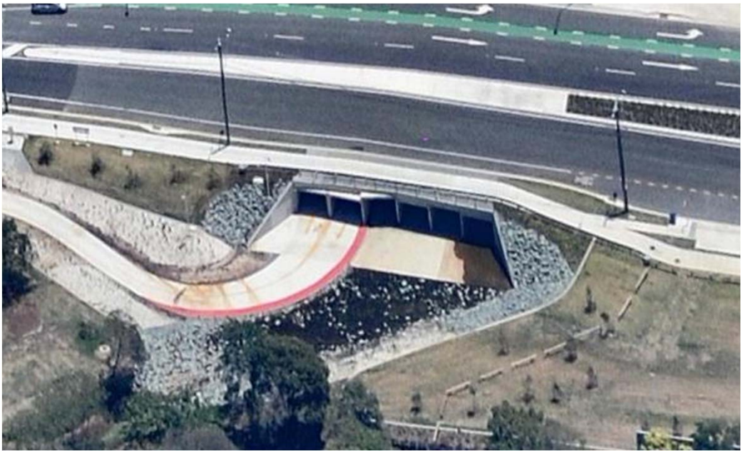
Robinson Road West looking downstream
