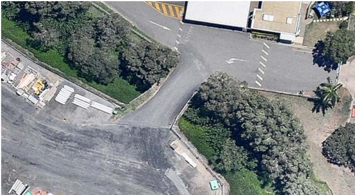
Culvert aerial view
