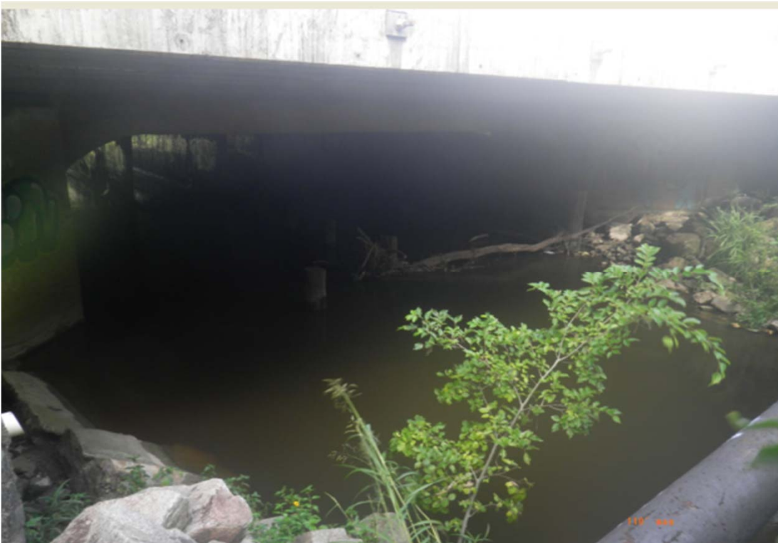
Gympie Road looking downstream
