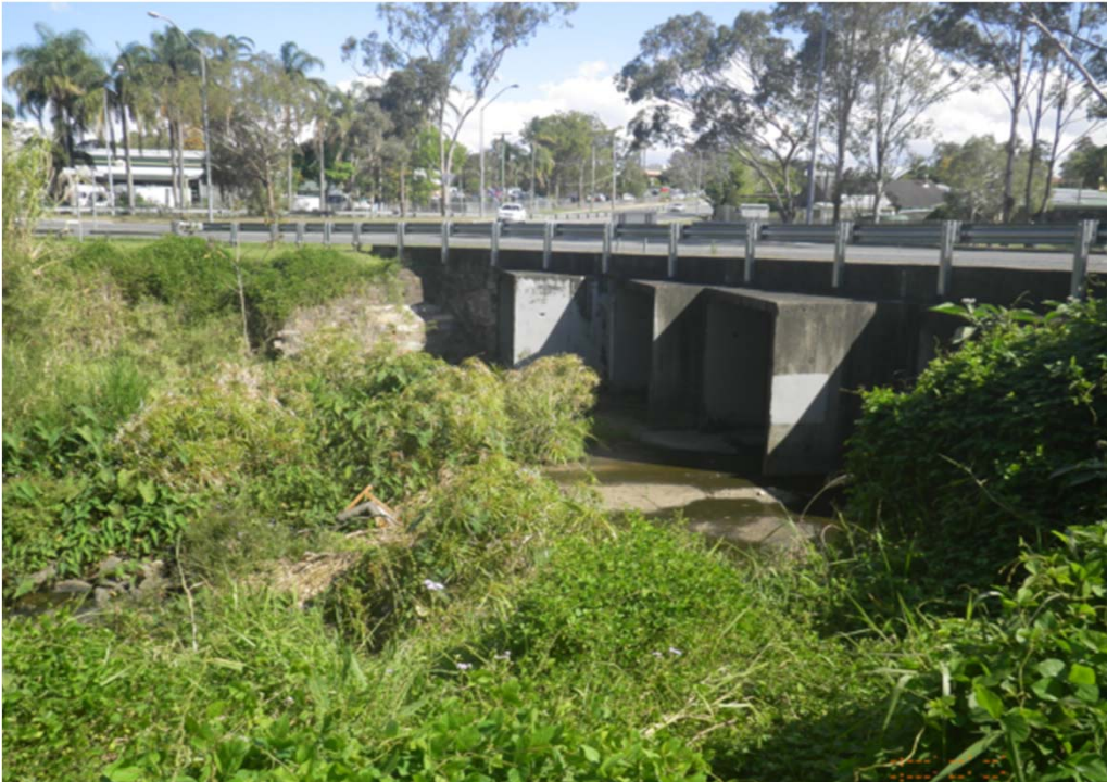
Culverts looking upstream
