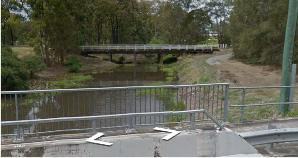
Bridge looking downstream
