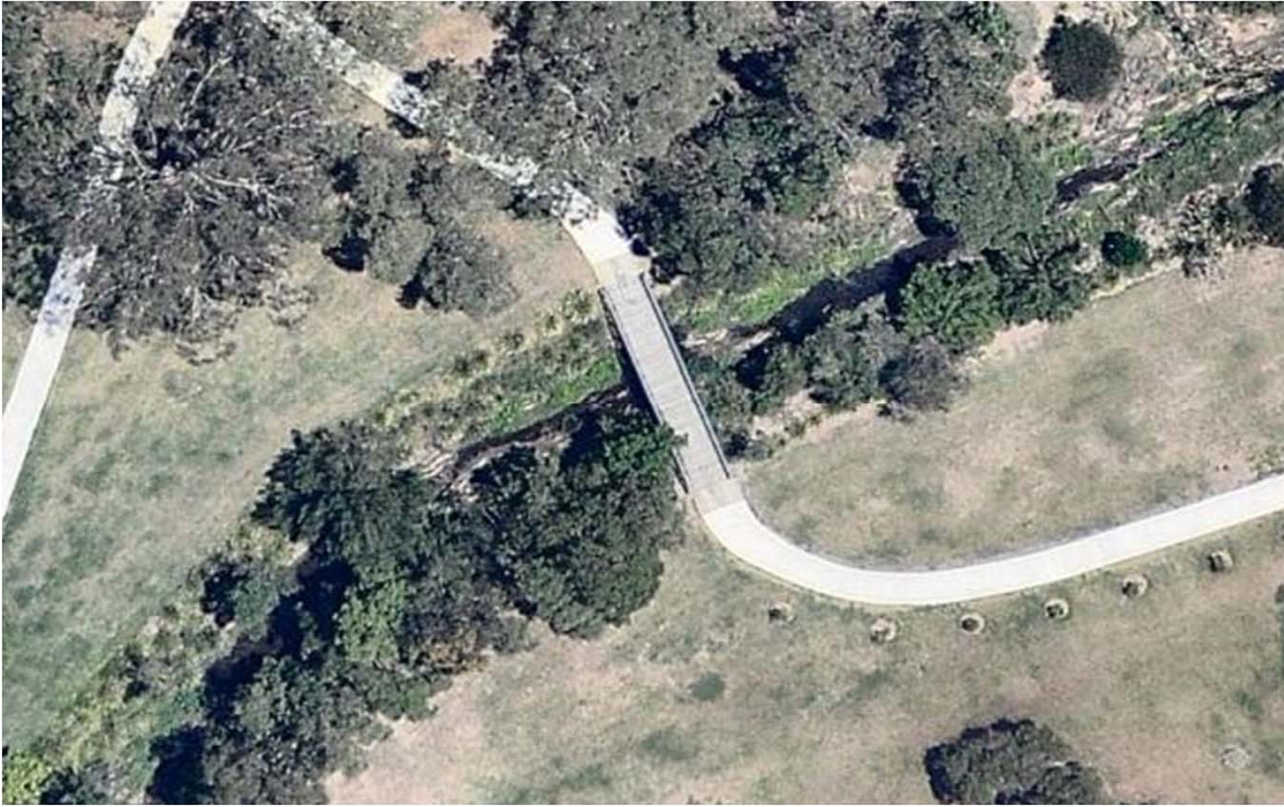
Rainbow Park footbridge aerial view
