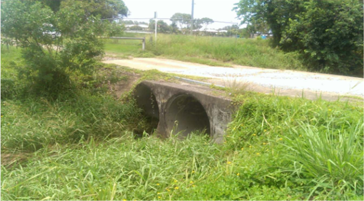
Culvert looking upstream
