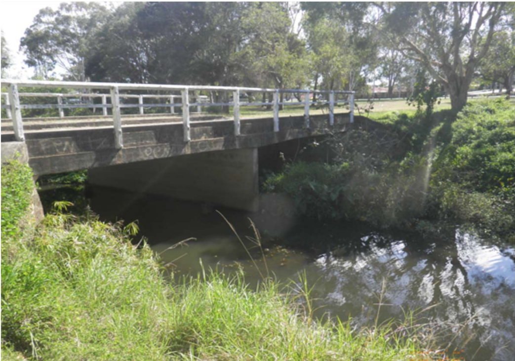
Bridge looking upstream
