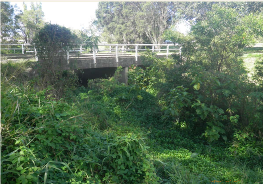
Bridge looking downstream
