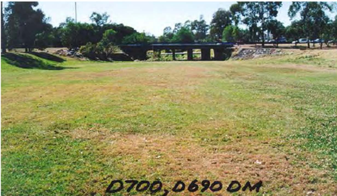
Culverts looking downstream
